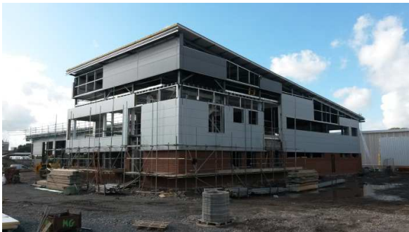
New Worcester Fire station under construction
